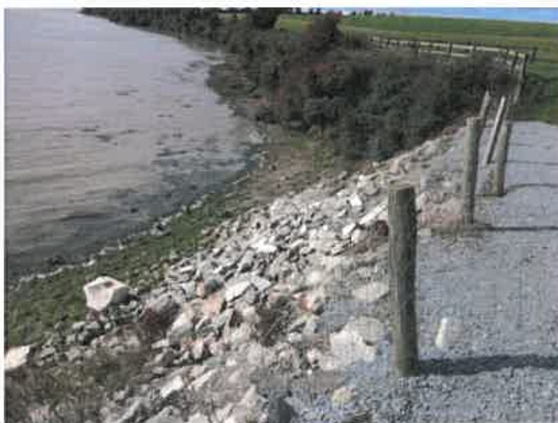
Large amounts of C&D waste material used for fill material within SAC and SPA for campervan parking
