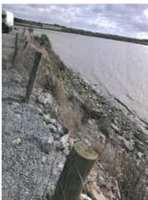
Large amounts of C&D waste material used for fill material within SAC and SPA for campervan parking
